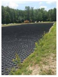
Installed in less than 4 hours, bags of discs were emptied into the basin and the cover immediately began serving as a bird deterrent, eliminating odors and keeping wildlife from coming in contact with potentially harmful deicing fluids.
