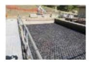
A solid cover presented safety issues, the discs did not. Summit Engineers was going to put aeration in these basins but saw a sample of the Hexa-Cover<sup>®</sup> product, called references then recommended the Hexa-Cover<sup>®</sup> installation. It penciled out better than aeration. That was important to this design build project, which Western Water Constructors, Inc. did with Summit.
