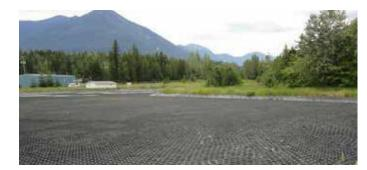
*"Familiar with the Hexa-Cover® Floating Cover, I felt the product could nicely cover the lagoon, controlling the algae growth as the sunlight would not be able to penetrate into the water. Additionally, the Hexa-Cover® Floating Cover would enable the aeration process and fluctuating water levels to continue"*
